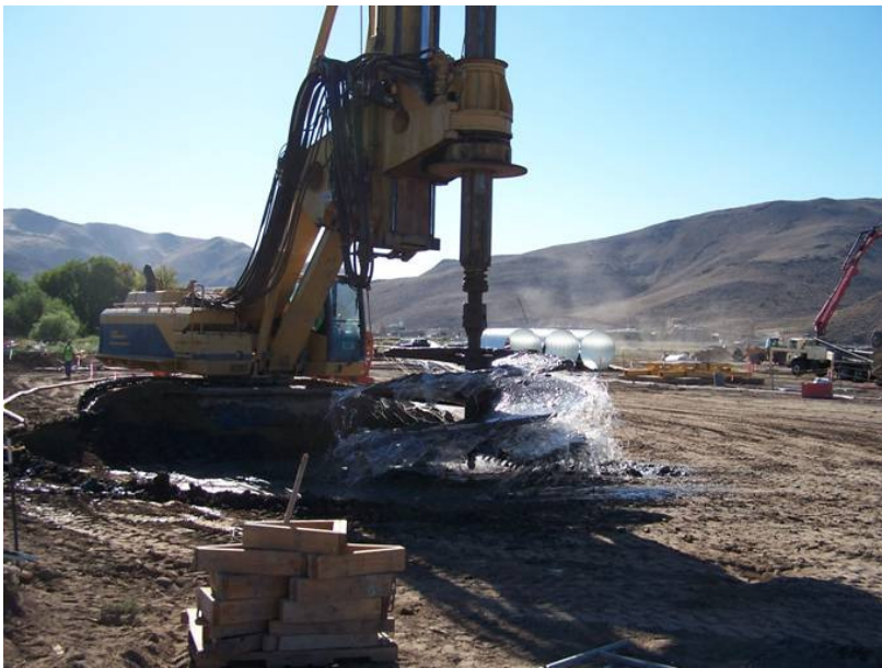
Drilling for a bridge support for the new southeast connector roadway
